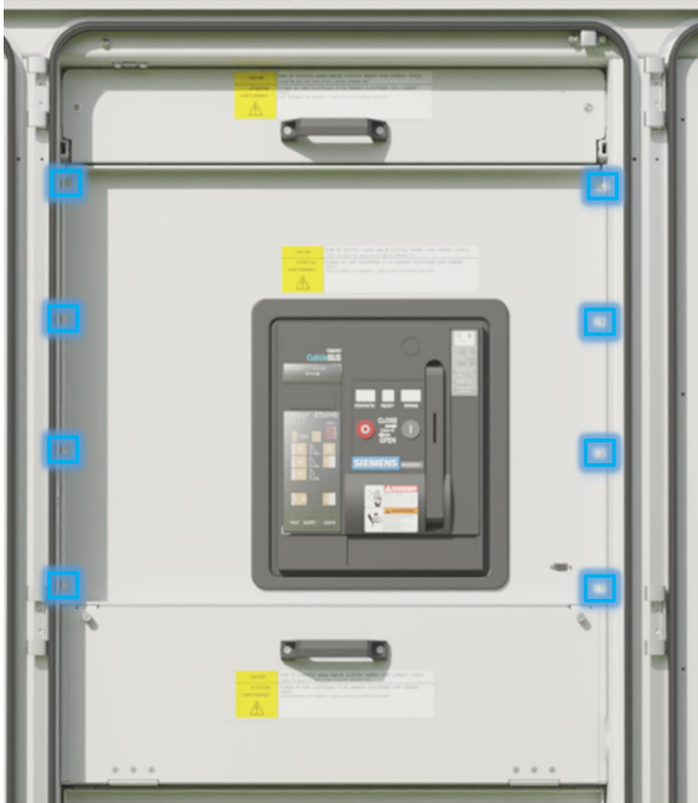
Figure 94. Removing Circuit Breaker Panel
