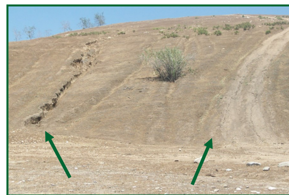
Hillside damage Hathaway Canyon, showing both an abandoned, rutted trail (left) and a new trail (right).
